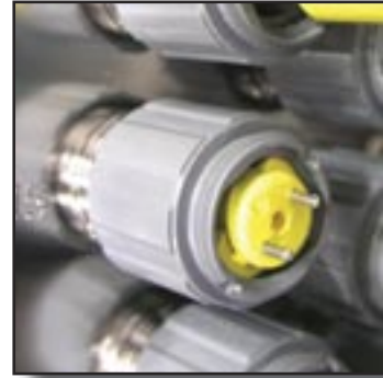
FIG. A INSERT LAMP INTO QUARTZ SLEEVE
