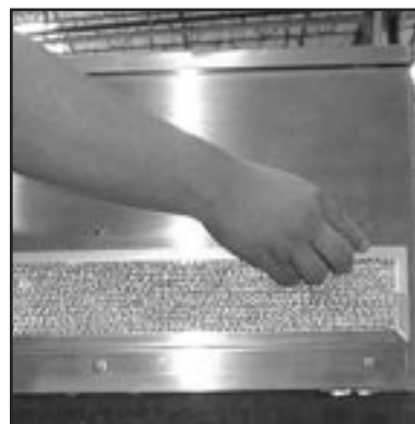
FIG. C LOCATE FILTER BY TOUCH
