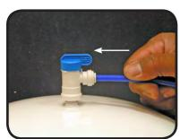
**Note:** Set the blue ball valve knob in-line with the blue tube, this is the "open" position.
