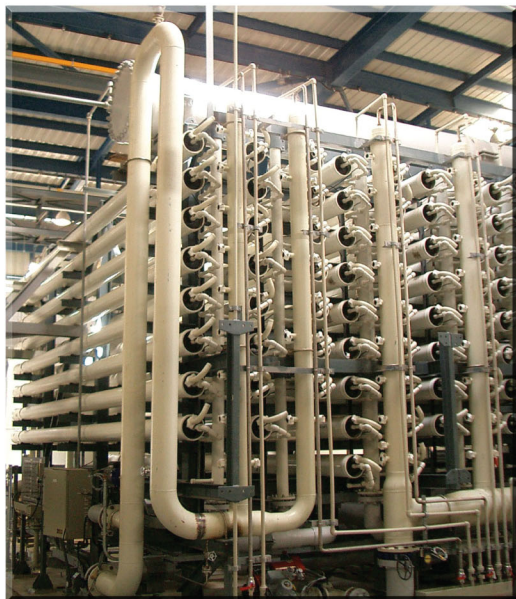
SWC membrane installation, 45 MGD (170,000 m³/d) in Fujairah, U.A.E.
