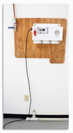
Step 2 Attach Water Processor at the upper and lower keyhole mounts. DO NOT PLUG IN.
