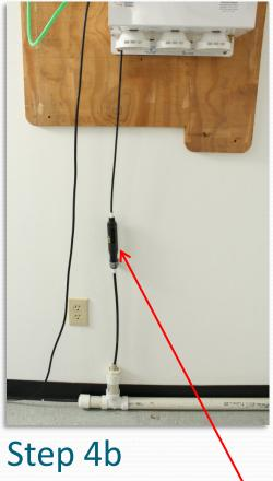
Connect Black Tubing from "D" Reject Water Outlet to an Approved Air Gap and Drain Line.
