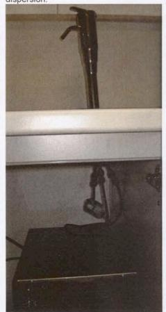
STEP 5 – Connect the faucet tubes to the water outlets in the back of the appliance, according to the labels.
