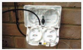
Typical use of a John Guest Gas Block/Fibre Lock & Straight Reducing Connector in a customer splicing point enclosure.
