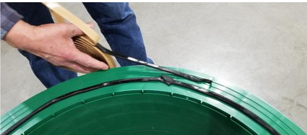
Apply the butyl to the BOTTOM of the TAR
