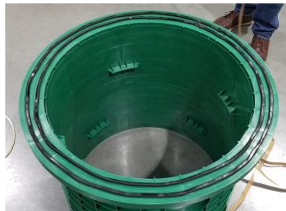
Firmly press the butyl to the TAR to form a full ring.
