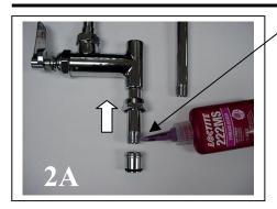
Install Nut onto base of Add-on Faucet & Apply Loctite 222 (or other non-permanent thread lock compound) to Add-on faucet's bottom threads.
