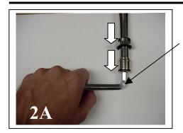
**Step 2A:** Using a 3/8" hex wrench, remove the bushing and locking nut from riser. (Either keep as spare parts or discard.)
