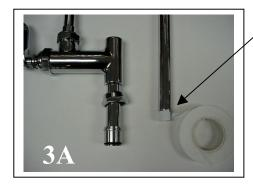
**Step 3A:** Apply plumber's tape or putty to base threads of riser.
